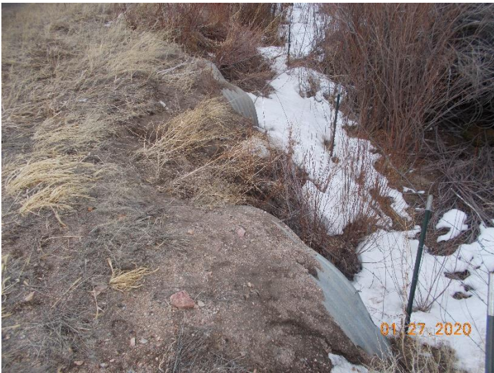
View of structure J-15-G looking southeast.
