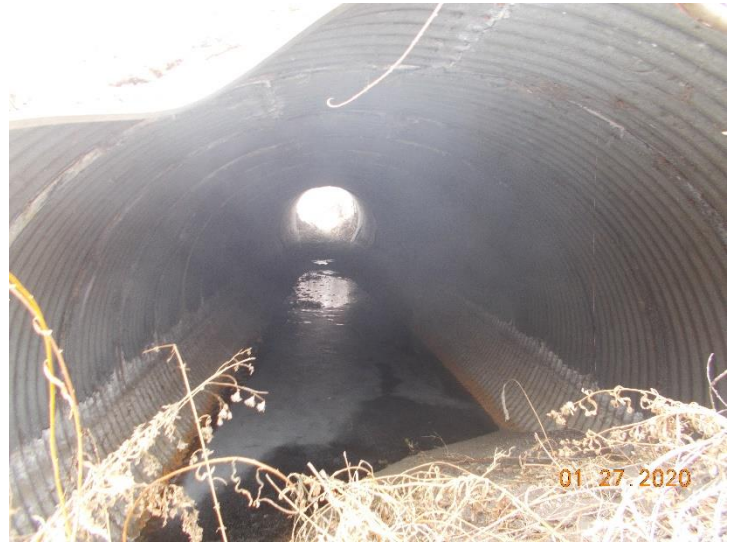
View inside structure J-15-G.
